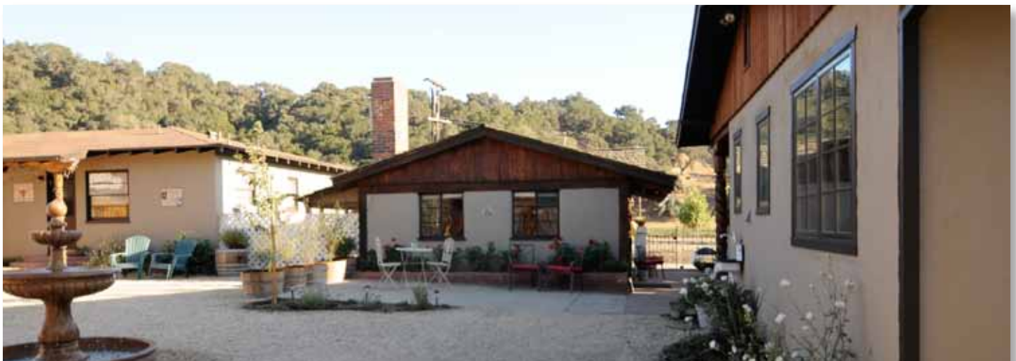
GUEST BUNGALOW LEFT, COOKHOUSE MIDDLE, REAR OF RETREAT HOUSE RIGHT. EDGE OF CONNECTING COURTYARD IN FOREGROUND.
